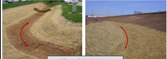
Channel Erosion Mat (duration of use, flow velocity, installation, maintenance)
