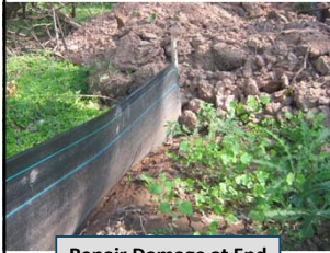
Repair Damage at End Of Each Work Day
