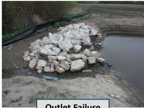
Outlet Failure
