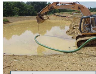
Sediment Trap or Basin (polymers to enhance settling?)
