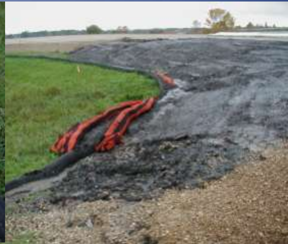
Channelized flow reinforced the bags
