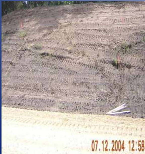
Ready for installation of compost blankets
